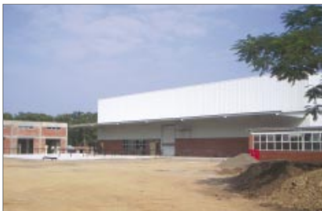
New facility in progress
